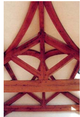
Exquisite detailing in the roof timbers
